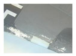
**Step 5:** Once the filler has dried, use fine sandpaper to smooth the repair. If you need to, apply more filler around the repair area to feather out the repair area.
